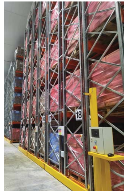
Lusaka Cold Storage.
